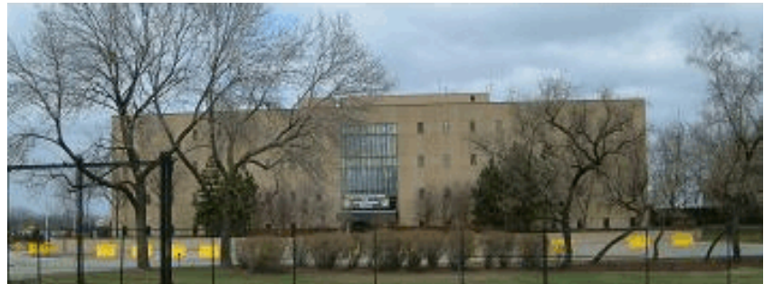
200,000 Square Foot TACOM Office Building #1
